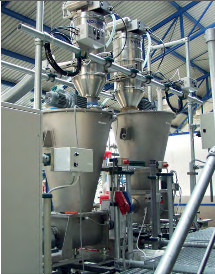
Two vacuum conveyors for loading loss-in-weight feeders.
